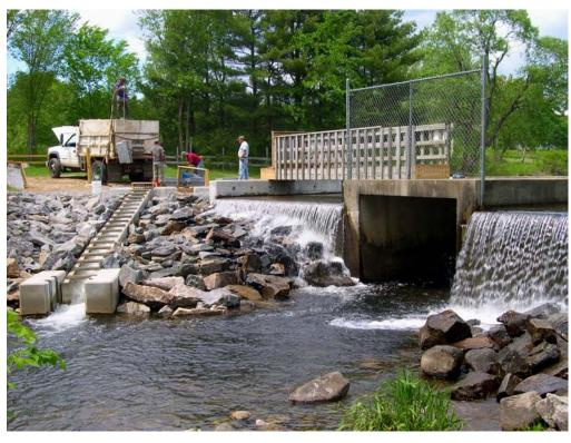
Clockwise from far left: The Benton Falls dam uses a fish lift to move spawning fish.
